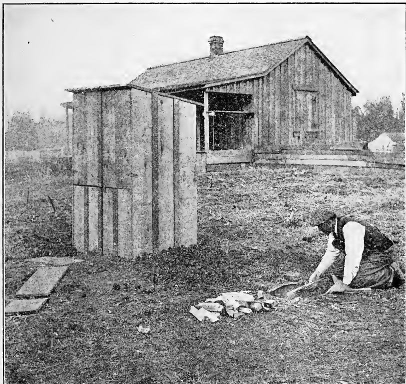
FIG. 2.—A smokehouse hastily constructed in the field. The operator is kindling a fire in the fire box, which, it should be noted, is several feet removed from the house but connected with it by an underground flue.
